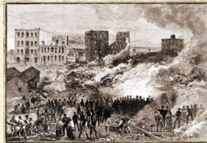
The Minneapolis Calamity, Debris of the "Washburn" and Two Other Mills in the Foreground -anonymous
